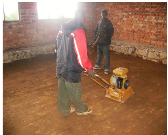
11 Compacting floor
