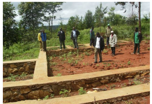
3 Authorities inspect foundation 2nd teacher house
