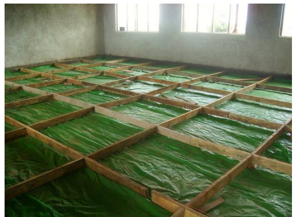
12 Preparing concrete tiles
