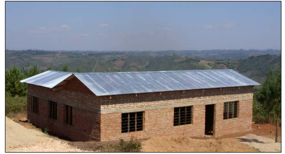
2 Head teacher house (windows & doors in progress)
