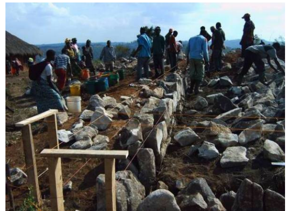
5 Constructing foundations
