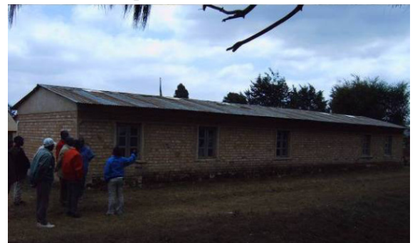
4 Existing school in main village
