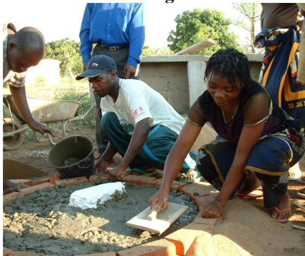
Picture 2 – Making a latrine slab
