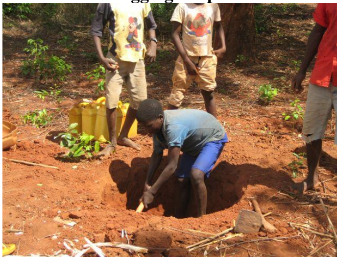
Picture 1 – Digging the pit of a latrine
