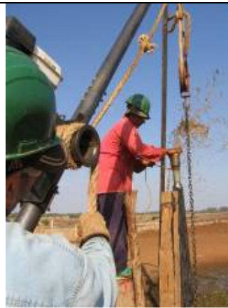
The drill bit is lifted with an engine
