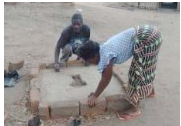
Husband and wife producing a latrine slab. (Ruaha village, Tanzania, 2006).
