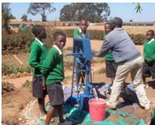
Borehole with rope pump at a school. (Njombe town, Tanzania, 2005).
