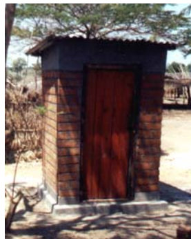
A finalized pit latrine. (Buza village, Malawi, 2002).
