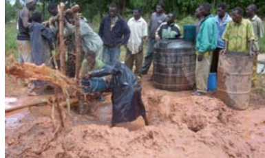
Rota sludge drilling in relatively soft soils in Njombe, Tanzania, can reach to 40 m. All labour is provided by beneficiaries. Three trained drillers supervise the drilling that takes 3 days on average.
