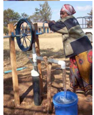
The rope pump is ready.
