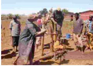
Rota sludge drilling in relatively soft soils in Njombe, Tanzania, can reach to 40 m. All labour is provided by beneficiaries. Three trained drillers supervise the drilling that takes 3 days on average.
